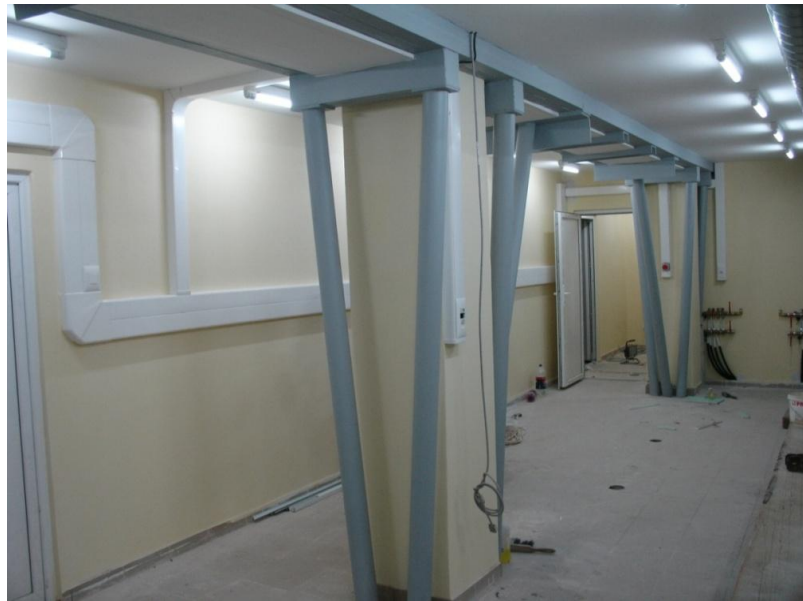
Fig. 12. Illustration of the load bearing structure reinforced by a steel frame
