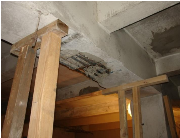
Fig. 5. Illustration of the propped up columns supporting the transverse beam
