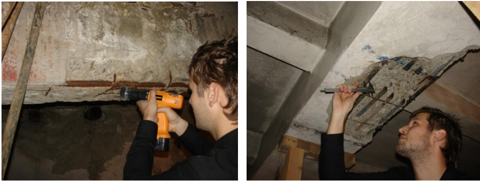
Fig. 9. Cleaning of reinforcement and consequent measurement of its diameter using a slide caliper
