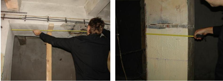
Fig. 7. Measuring the dimensions of particular structural elements of reinforced concrete frame
