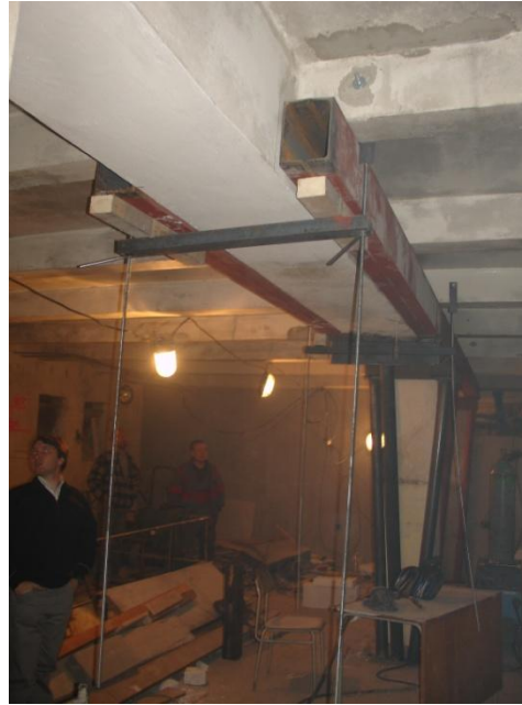
Fig. 11. Process of installing the steel construction
