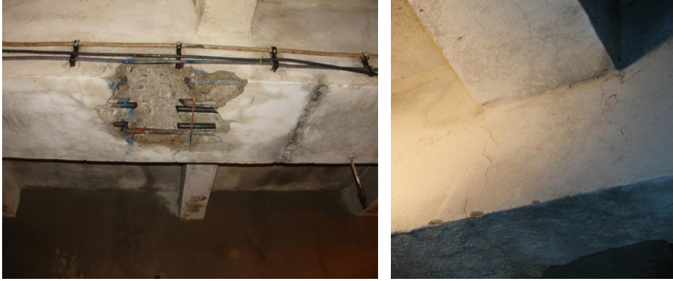
Fig. 3. Illustration of the compromised (cut) reinforcements of the transverse beam
