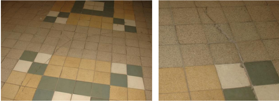
Fig. 4. Illustration of the cracked floor above a part of the ceiling which was subjected to damage from failure in the transverse beam
