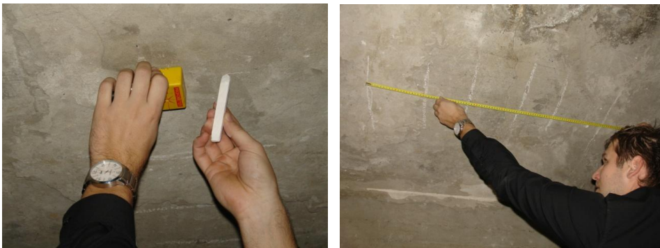
Fig. 10. Position and marking of the reinforcement on the flooring plate of the ceiling using a magnetic indicator – Profometer
