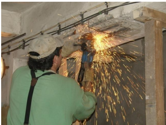
Fig. 12. Restoring the load bearing capacity of the beam by welding and rejoining the cut reinforcement
