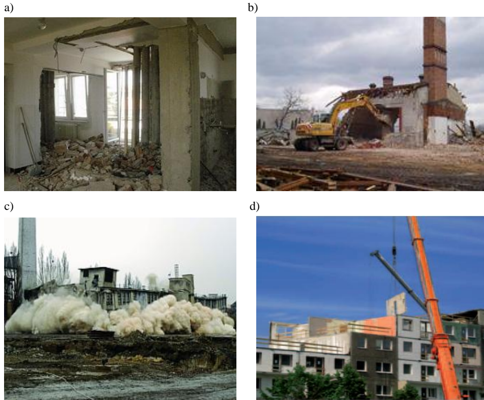
Fig. 1. Demolition and deconstruction of building structures: a) manual demolition of structures, b) demolitions through the mechanization, c) demolition of construction by explosion, d) deconstruction of structures
