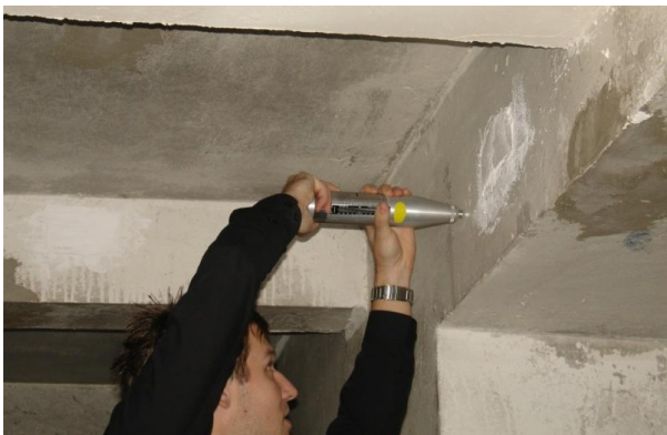
Fig. 8. Non-destructive method of determining concrete strength by means of Schmidt impact hammer tests
