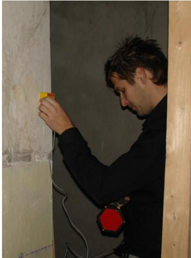
Fig. 11. Position and marking of the reinforcement in the frame and in the transverse beam using a magnetic indicator – Profometer
