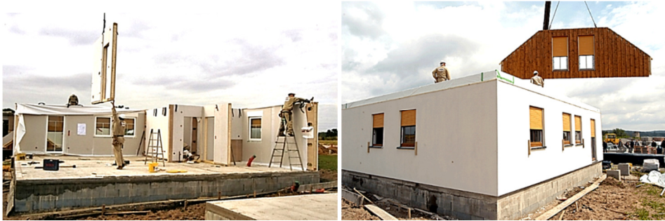
Fig. 2. Construction of panel construction system [12]
