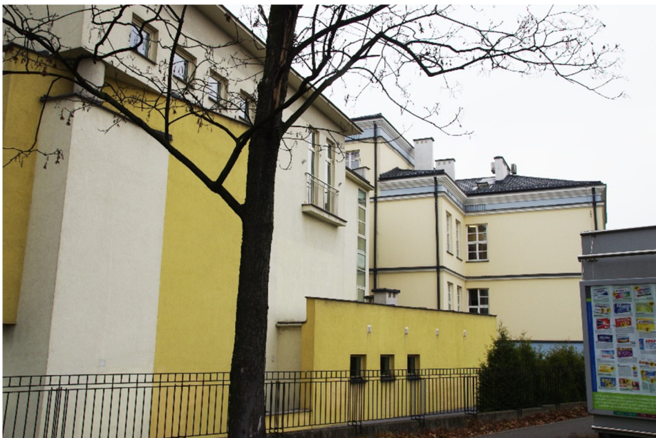
Fig. 3. View from Ciepliński Avenue before the design process shows the chaotic form of analyzed building. Source: Archive of MWM Building Design Group design studio, Rzeszów, Poland
