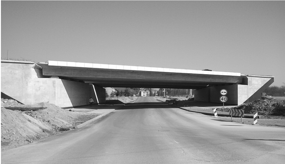
Fig. 1. The viaduct WA-164 A4 motorway
