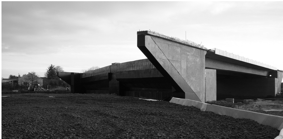
Fig. 4. View on the viaduct before backfilling the abutments
