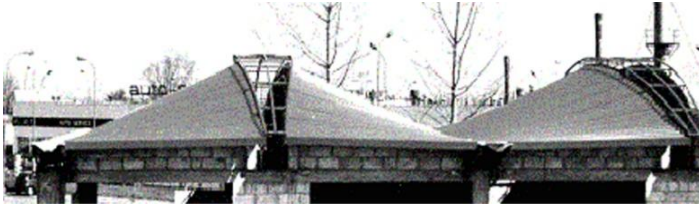
Fig. 1. The multi-segment shell structure [2]
