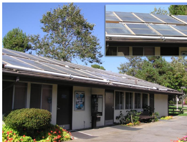
Fig. 2. Laundry supplied by solar power
