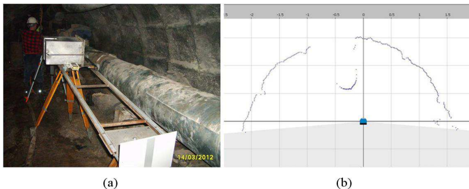
Fig. 8. The laser mining scanner in a self-propelled layout (a) and a single transverse scan of the excavation (b)
