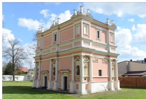
Fig. 2. The view of Loreto Chapel from the south-west (Author's picture)
