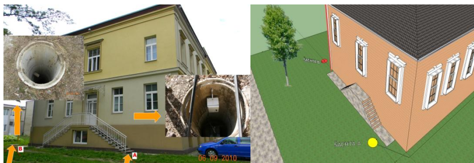
Fig. 5. Location of infiltration shafts near building PK6
