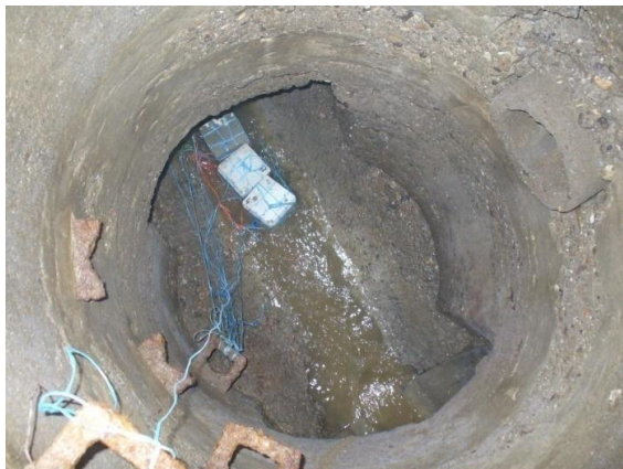
Fig. 1 Concrete samples placed into the sewer system of Kosice city
