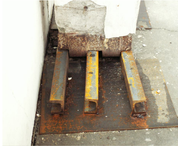
Fig.13. View of column after being wedged up with steel profiles
