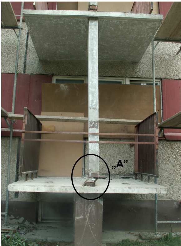
Fig.2. Ground floor column after stability loss
