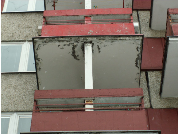
Fig.4. View of corrosion damage of structural elements of balconies
