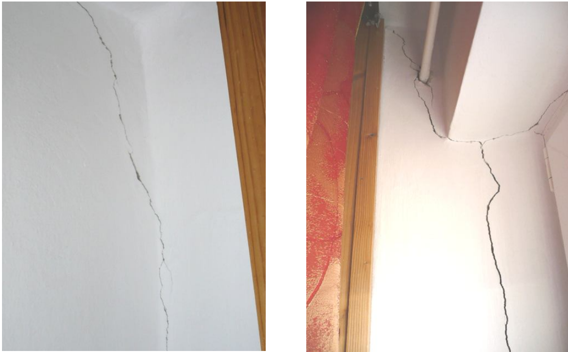
Fig.10. Cracks at wall connections
