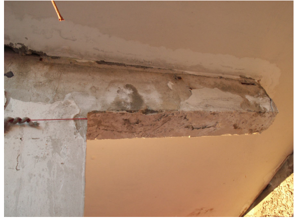
Fig.5. Corrosion damage of cantilever beam supporting balcony plate
