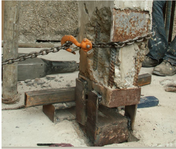
Fig.12. Column of supporting structure of balcony immediately after plumbing
