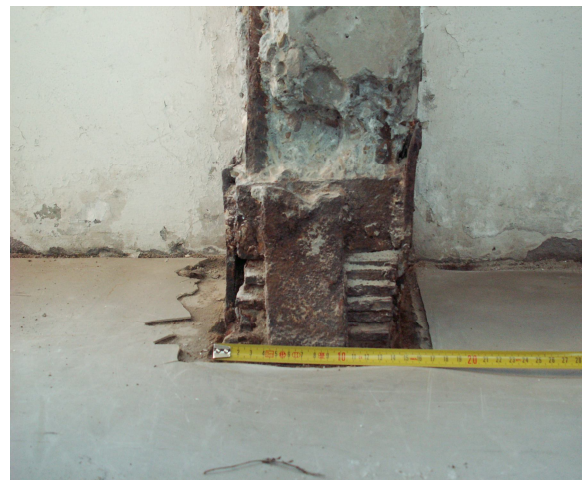
Fig.7. Filling between balcony slab and column base
