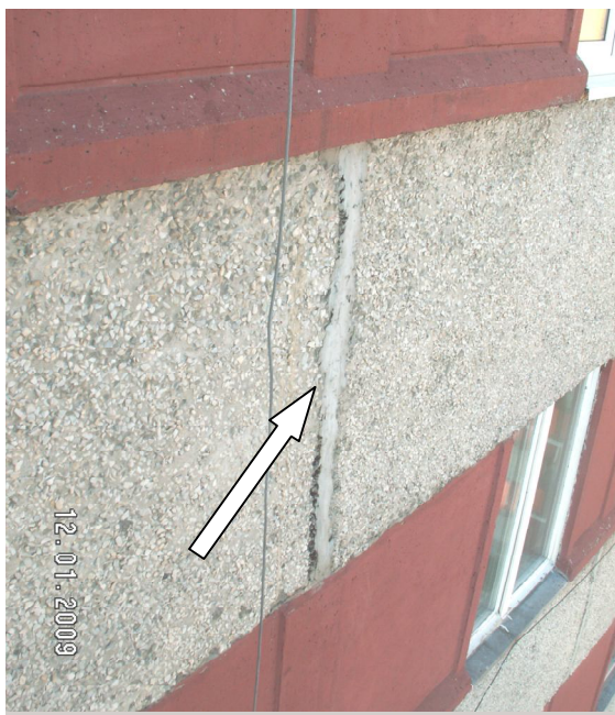
Fig.8. View of displacement (~ 20 mm) of facade plate of the highest storey
