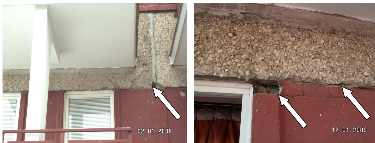
Fig.11. Damage to facade plates
