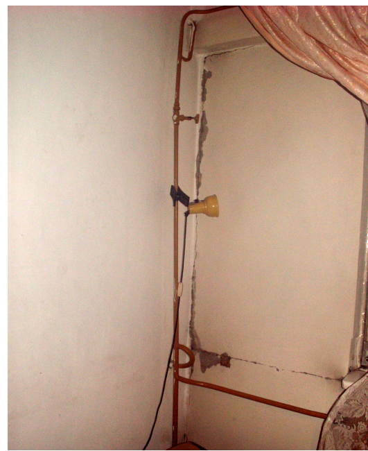
Fig.9. View of façade wall displaced from inside
