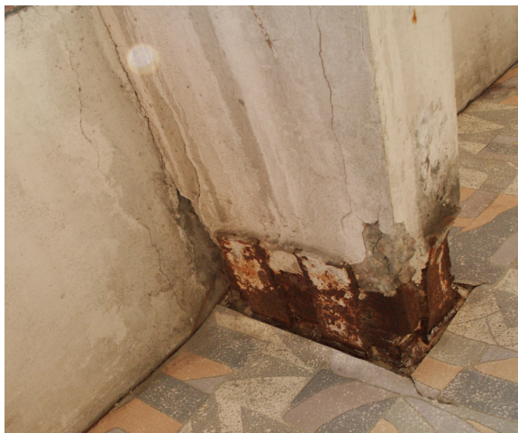
Fig.6. Corrosion damage of column base
