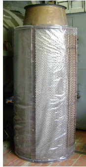
Fig. 1. Overview of cylindrical filter air distributor
