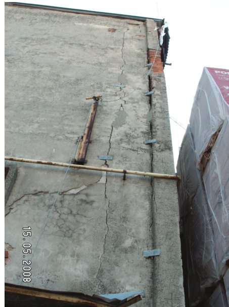
Fig.7. Gable wall, corner A-0 – damage and separated strata along longitudinal wall
