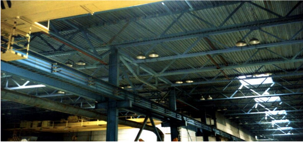
Fig.5. Truss beam-girder L=12\text{m} . Experimental research factory, Lviv, 2004.
