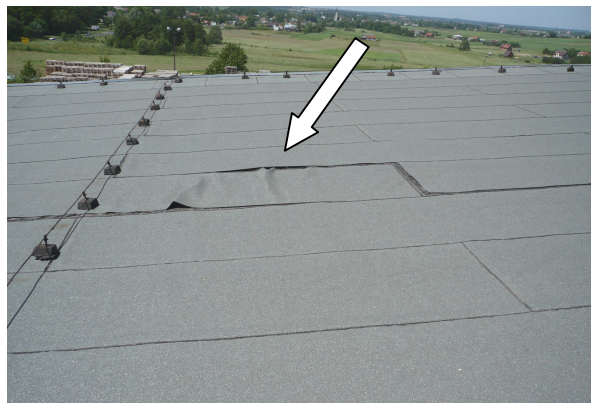
Fig. 5. Hollow in roof at slab slip-off
