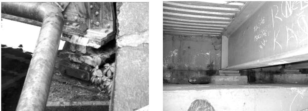
Fig.4. Improper bearing details
