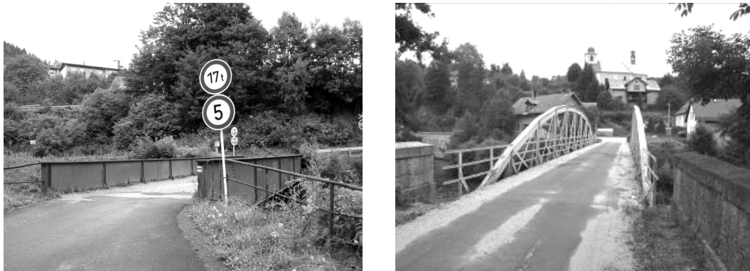
Fig.5. Bridge in Jablonec erected in 1883 (left), Bridge in Haje erected in 1872 (right)
