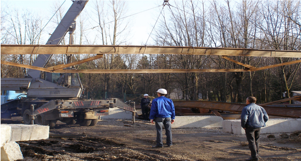
Fig.2. Erection of low element sub diagonal girder with span L=12 m. Sanatorium "Zeneva" Truskavez, 2004.
