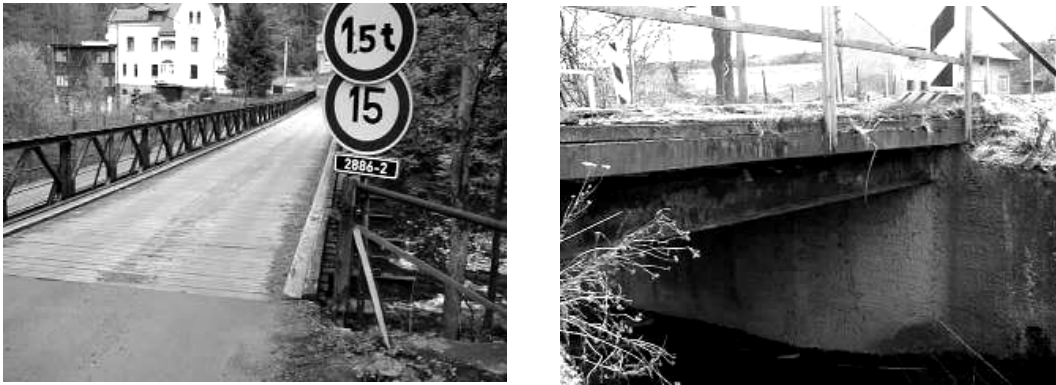
Fig.6. Bridge in Rusalka erected in 1948 (left), Bridge in Kokovice erected in 1961 (right)
