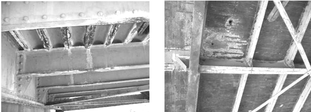
Fig.3. Deck slab corrosion
