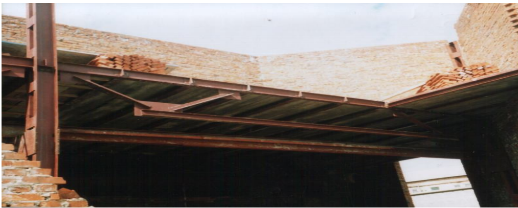
Fig.6. Beam-girder of floor
