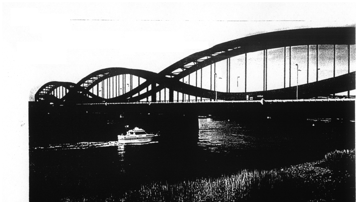
Fig. 3 The Bridge in Hamburg (1887 – Germany) created by three funicular spans of L = 100\text{m} called as “fish shape”. The stiff short column acts as the hoisted support in axis for simple spans. The axial horizontal railway is partly supported by studs and partly suspended on the hangers.
