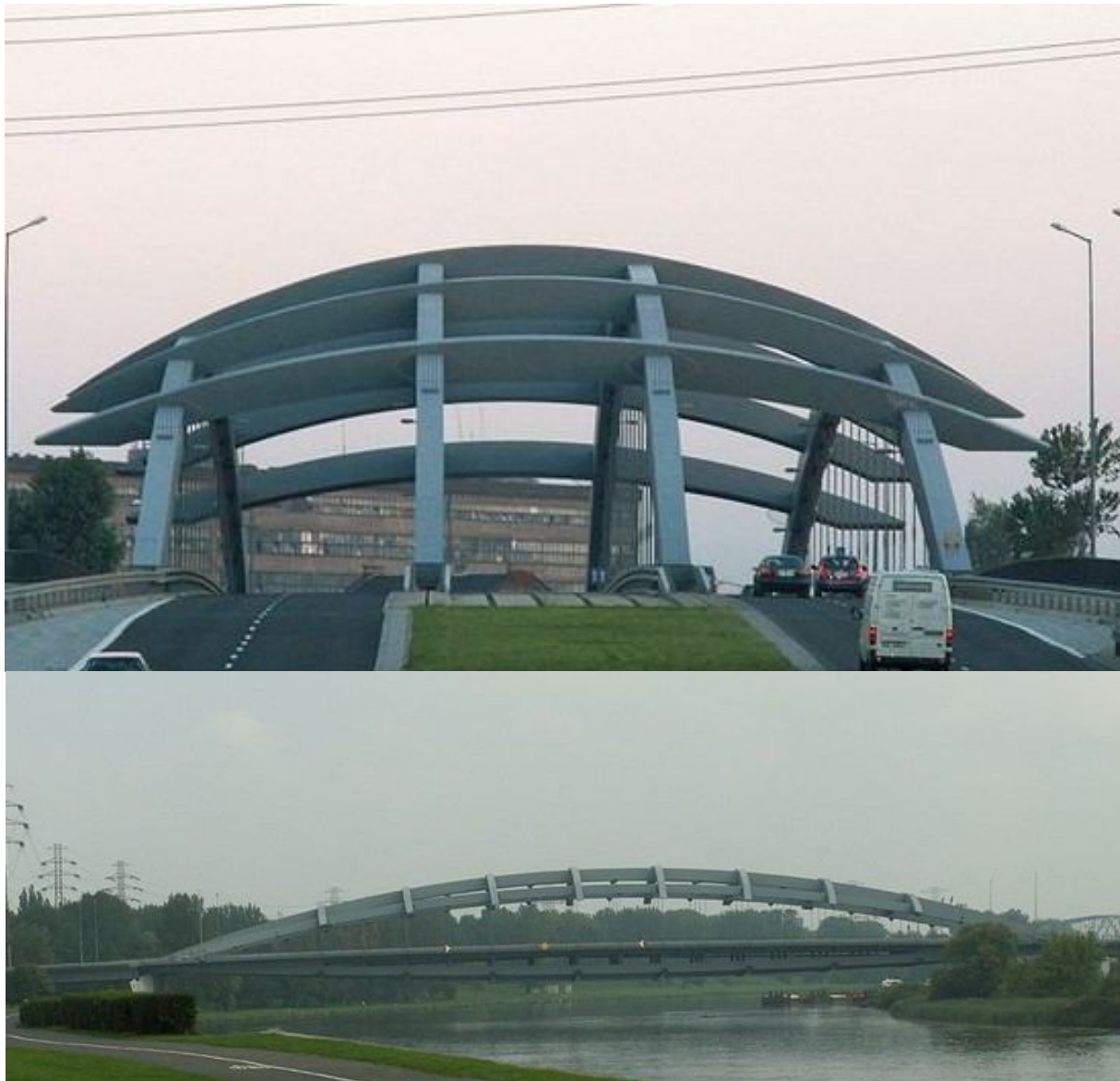
Fig. 4 The Kotlarski Bridge in Cracow ( Poland ), span L = 166\text{m} , build 2004.
