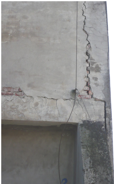
Fig.6. Separation of gable wall in axis "0" from longitudinal wall in axis "B"
