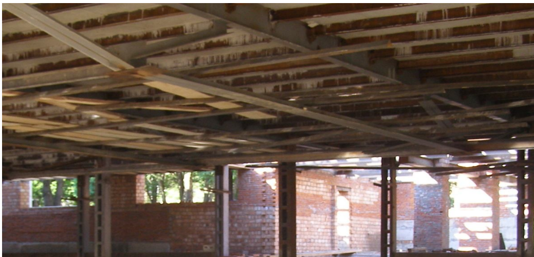
Fig.3. Appearance of beam-girder under construction L=18 m. Sanatorium "Zeneva" Truskavez, 2007.
