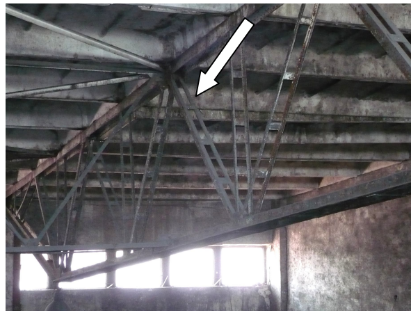
Fig. 3. View of roof slabs off the girder in axis 1
