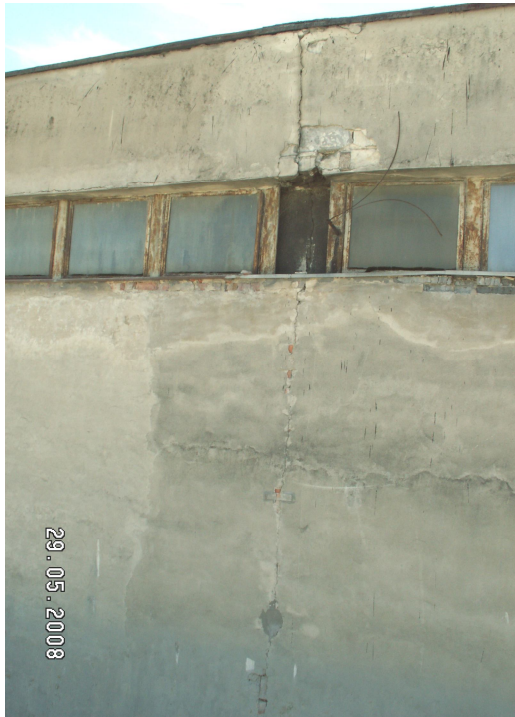
Fig.10. Wall in axis “B”. Dilatation between axes 15 – 15’- general view
