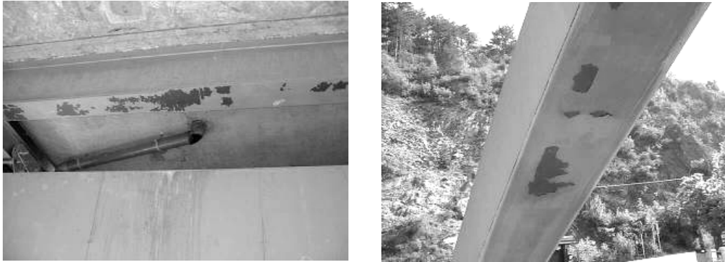
Fig.1. Defects of protective coating
