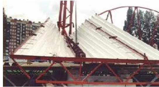
Fig. 13. The deformed shell sheets [2]
