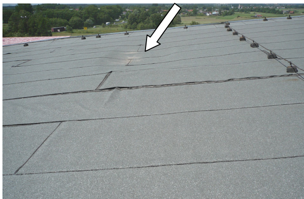
Fig. 4. View of roof slabs off the girder in axis 1
