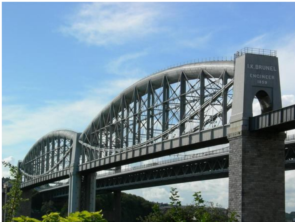
Fig. 2 The Saltash Bridge (England) designed by Isambard Kingdom Brunel as funicular truss, (1859) with 2 chords.
