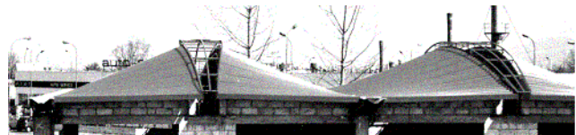
Fig.2. Building shell made up of the flat sheets deformed in the planned way [2]
