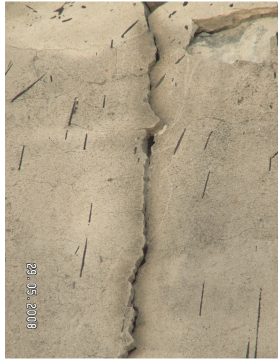
Fig.11. Detail “b” – wall parts displaced relative to each other
