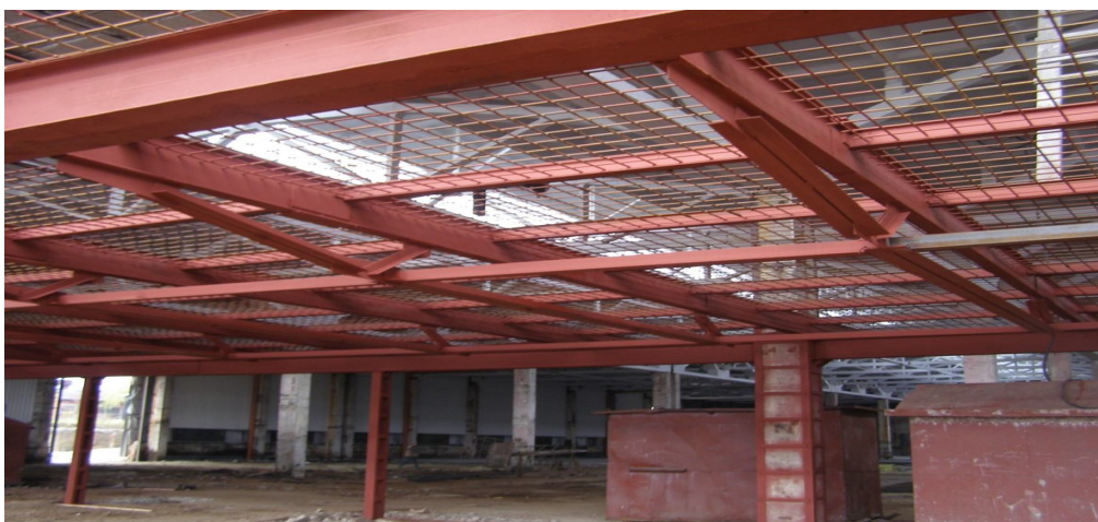
Fig.4. Light combined girders of floors with effort regulation. L=12 m. business center "Pidzamze" Lviv, 2007.
