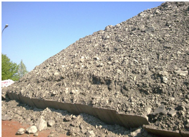
Fig. 2. Dump after losing slope stability
